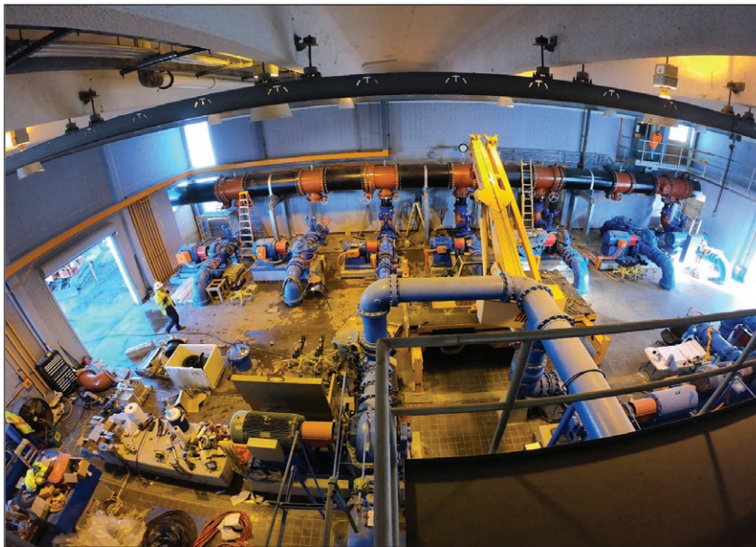
Figure 14. Phase 3 – Tie-in of pumps to header.
