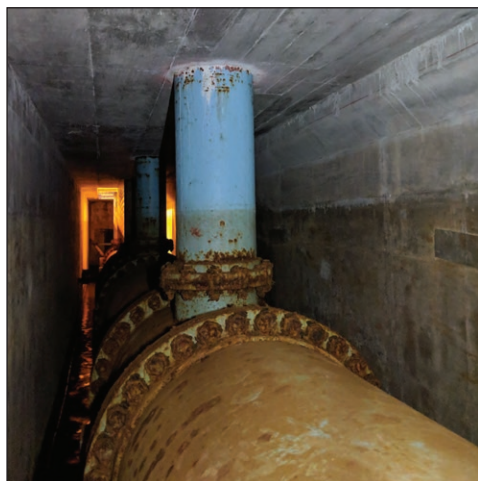
Figure 1. Discharge header pipe tunnel.
