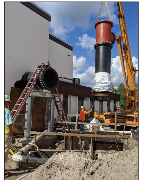
Figure 16. Phase 4 – Eastern tie-in.
