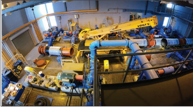
Figure 12. Phase 2 – Beginning of header pipe construction.
