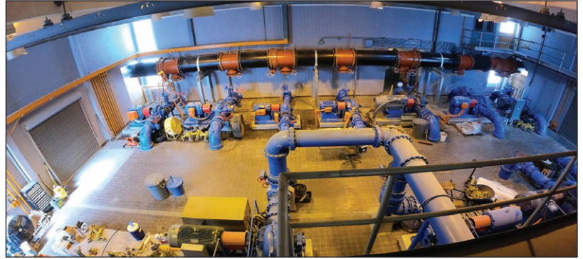
Figure 13. Phase 2 – Header pipe construction.
