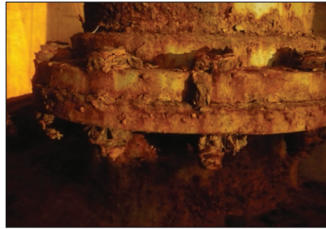
Figure 3. Corroded flange and bolts from a high-service pipe into a header.
