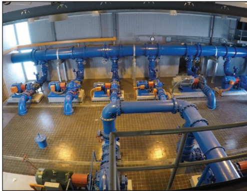
Figure 17. Phase 5 – Completion of the project.
