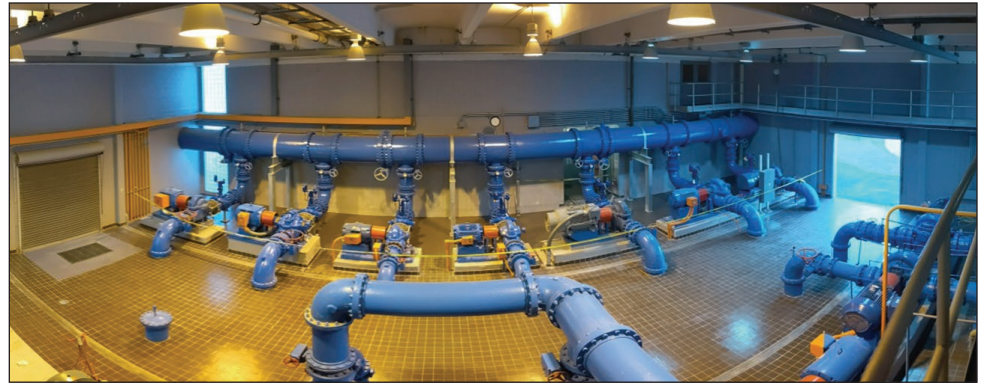
Figure 18. Phase 5 – Completion of the project (full view).
