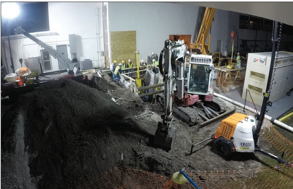
Figure 15. Phase 3 – Line stop at west discharge point.
