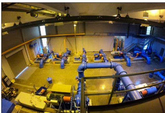
Figure 9. High-service pump station pump room prior to construction.
